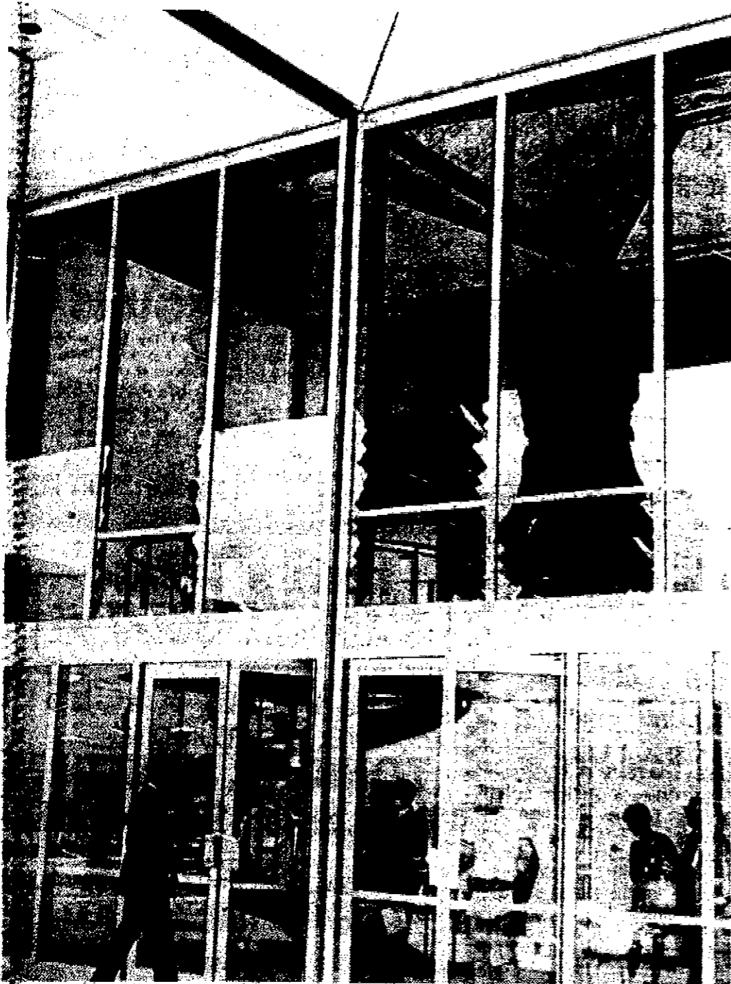
NORTH ENTRANCE, MITCHELL HALL — Several persons who were watching the ceremonies at this entrance to Mitchell Hall were cut by flying glass. Academy Chaplain Roy Terry, who was standing on the second floor, near the railing behind the third window from the right, escaped injury.
