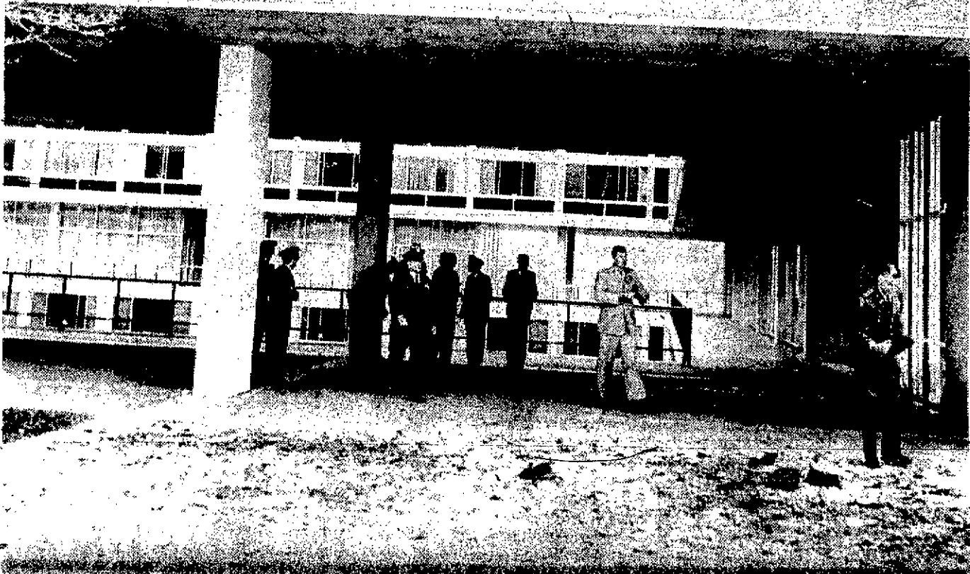
THE AFTERMATH — This was part of the aftermath of a sonic boom at the Air Force Academy caused by a low-flying F-105 jet, one of four, which was to fly over at the climax of ceremonies presenting an F-105 for permanent display at the academy. This is some of the damage to Vandenberg Hall, a cadet dormitory. At lower right, one of the men whose hats were knocked off by the shock wave and who were caught in a shower of glass tries to reclaim his property. (Gazette Telegraph Photo)
